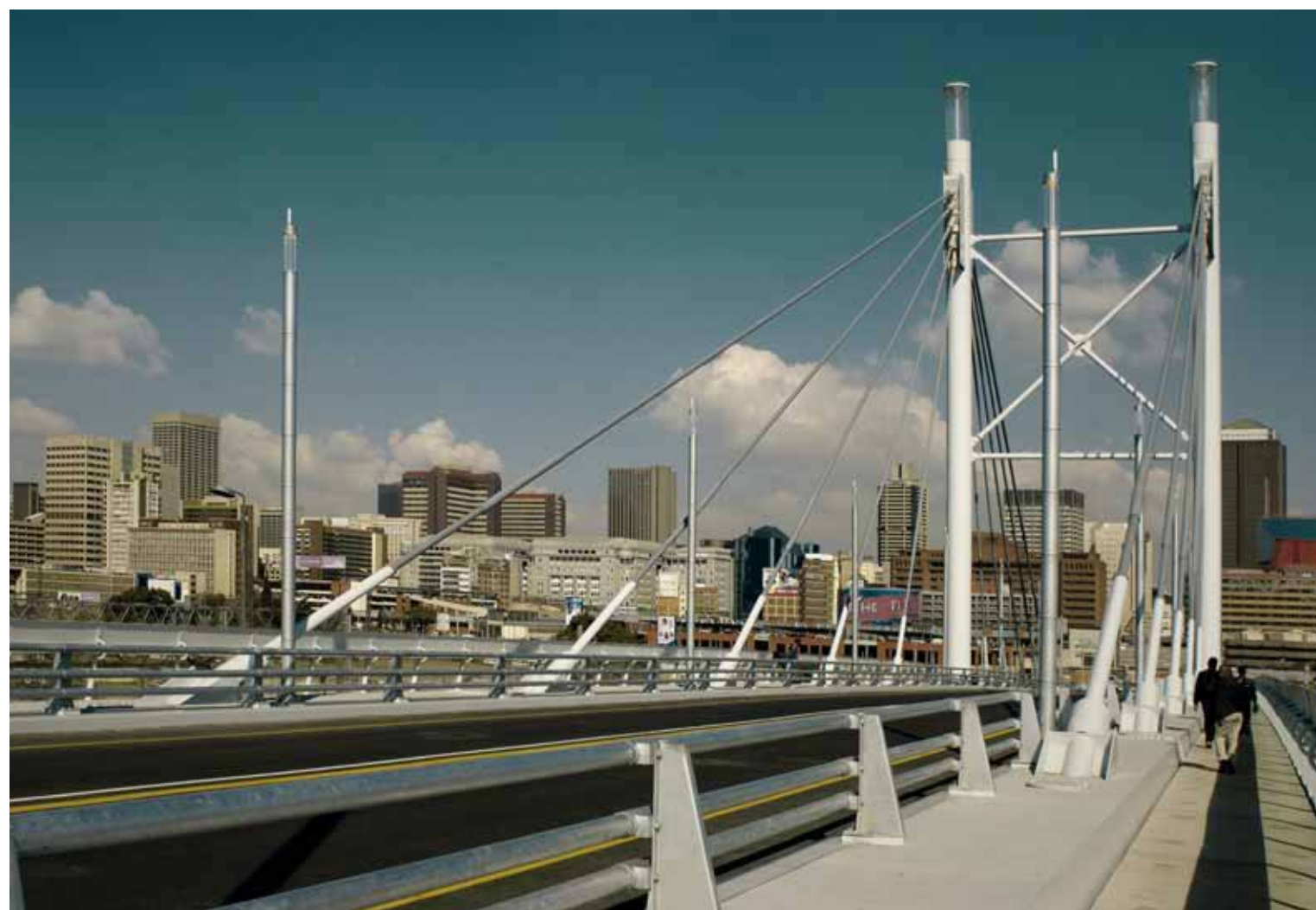
Nelson Mandela Bridge, Johannesburg
